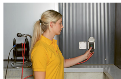
3 Mobiler FI-Schutz (RCD)
