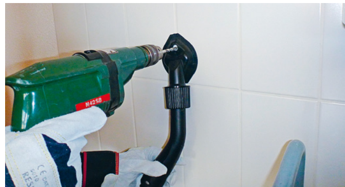
Loch in Platte bohren
