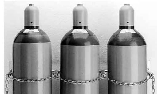
Fig. 1: Securing compressed gas cylinders with chains.
