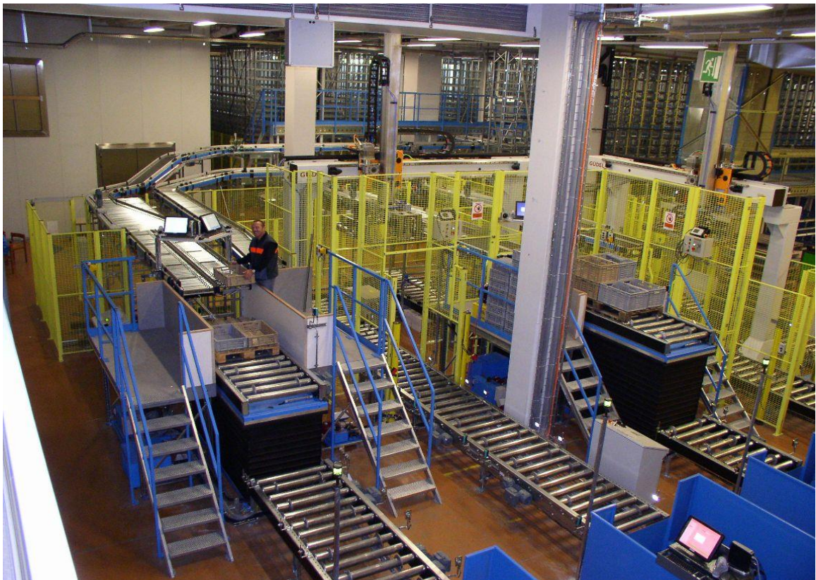
Fig. 3: Same plant as in Fig. 1, here prior to commissioning
