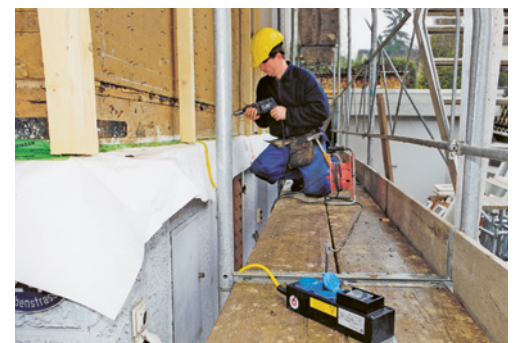
8 If no worksite distribution board is present: use mobile residual current device (RCD).
